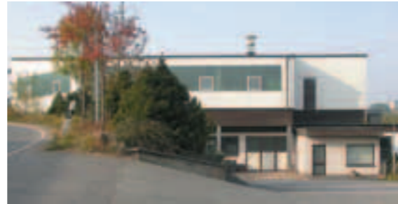
Front side of the business premises
